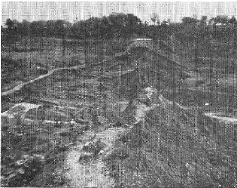
Photo. 8 Dam destruction of Hayakake-numa Reservoir
