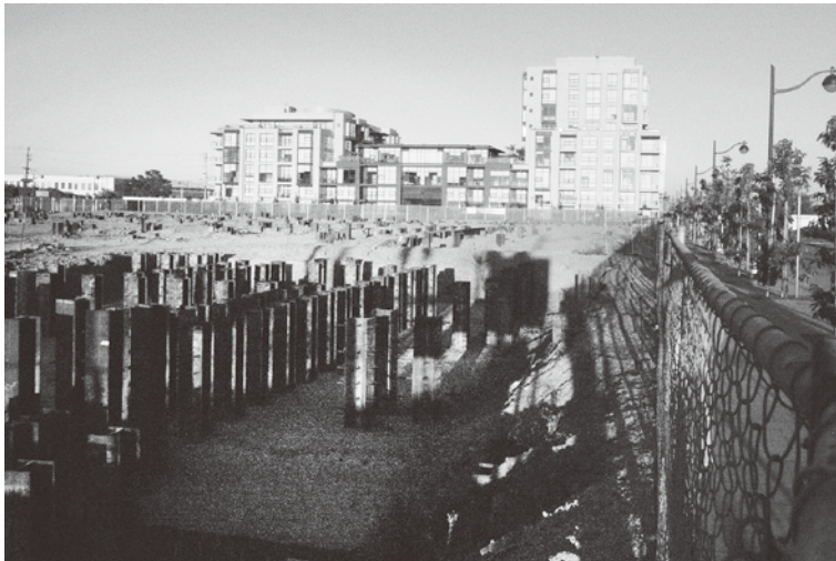
Photo 1 On-going Mission Bay redevelopment Photograph by Takashi Oda, in October 2008
