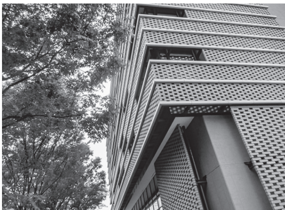
Fig.5 Seinan Gakuin University Library (New construction)
