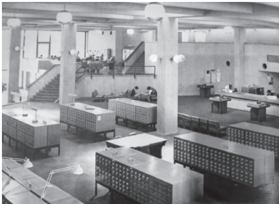
Fig.12 Main Area (New Construction)
