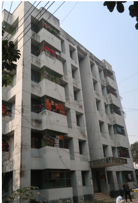
6.25 General view of the surveyed building no 3
