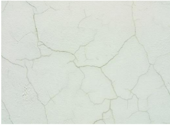
(a) Plaster crack ( do not consider)
