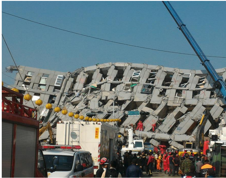
Figure 2.14 Severely damaged buildings in Taiwan earthquake (datacenterhub.org)
