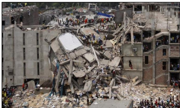
(a) Rana plaza collapse
