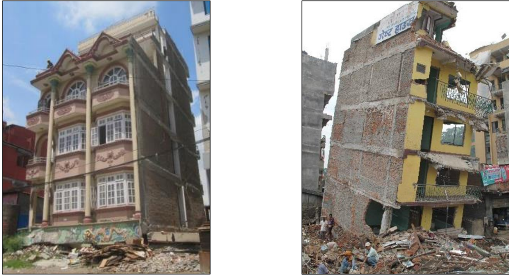
Figure 5.5 Examples of buildings subjected to soft-story collapse during the Nepal earthquake (datacenterhub.org)
