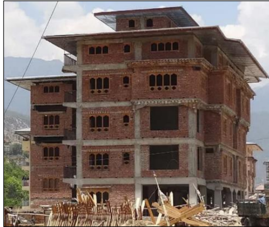
Figure 1.2 Building with Masonry infill (Photo: Janise Rodgers, Bhutan)
