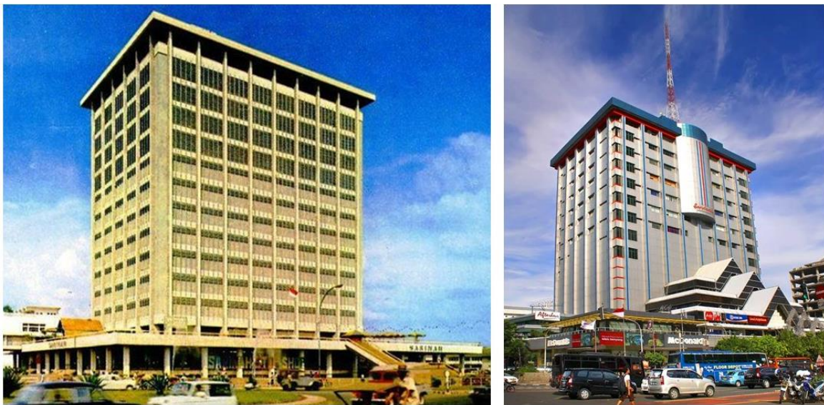
Figure 4.3 The change of façade of Sarinah Department Store, where the 1960s original design (left) covered with ‘colourful’ cladding and three layers of gable roof as the hat of its podium in 1990s (right) (source: https://3.bp.blogspot.com/-kqI5SGvG-Lo/WNU3rNOFTxl/AAAAAAAAAKY/sPIlrL3VtVod3zQYM5nTDLcdUKgD1P3ugCLcB/s1600/gedung-sarinah-tempo-dulu.jpg accessed April 7 2016 (left), https://mapio.net/images-p/90351641.jpg accessed April 7, 2016 (right))
