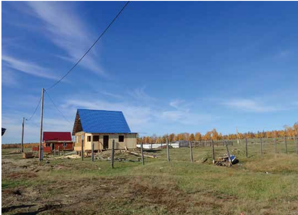
Fig. 8-4: Residential building with an embankment at the base (photo by Y. Fujioka, Churapchinsky District, 2016).
