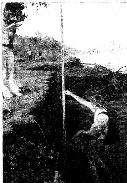
Photo 1 Erosion along the coast in Rajekwesi village, Banyuwagi, Java.
